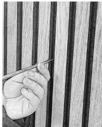
⑤ Nail the upper wall
