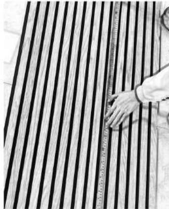
② Measure the wooden slat acoustic panel
